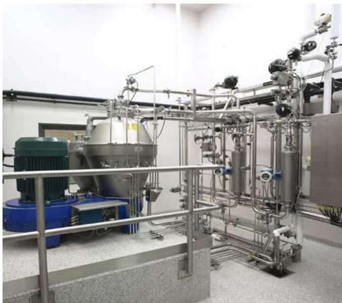
Figure 10-32. A centrifuge, pump, motor and associated piping
